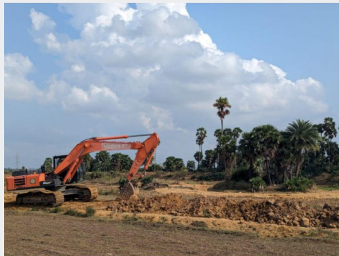
Periphery embankment creation
