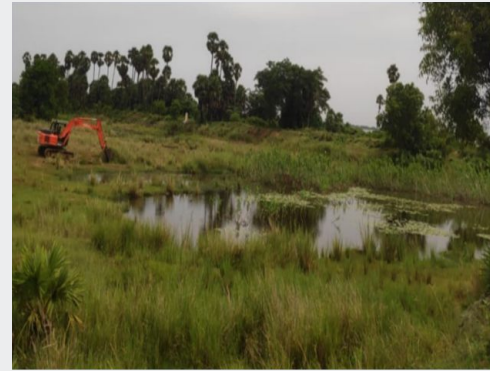
Removal of the weeds and shrubs
